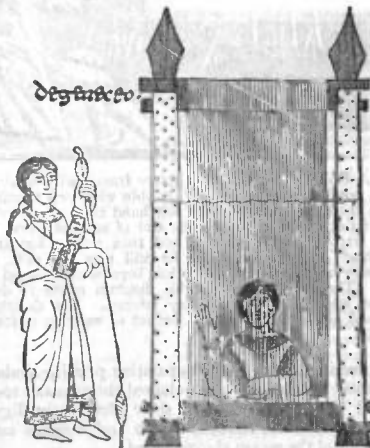
FIG. 4.—High warp frame from MS. Codex by Rabanus Maurus (9th century).
